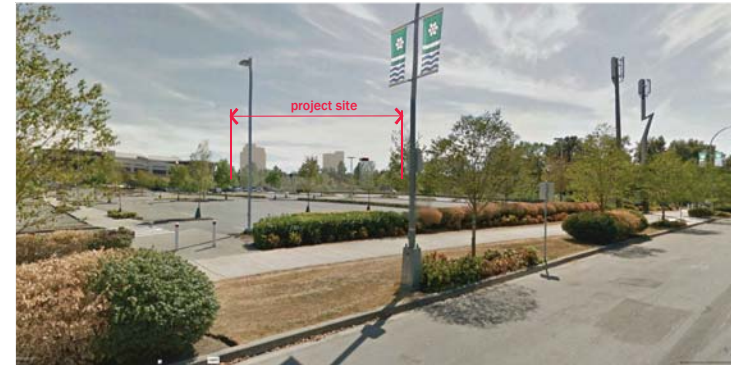
2 200th Street & 80th Ave - View Looking Southwest
