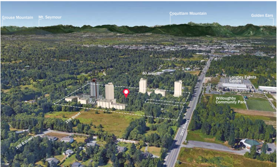
Aerial View Looking Northwest
