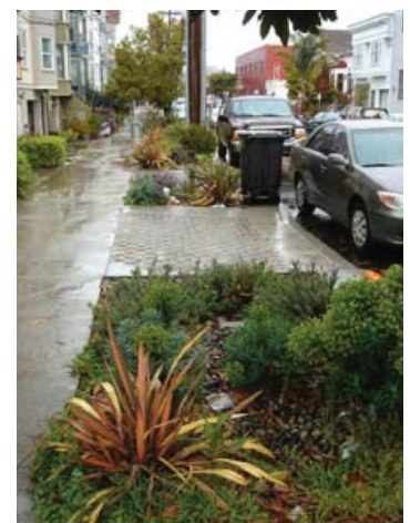
Figure 80. Storm water source controls like these rain gardens reduce pollutant run-off.
