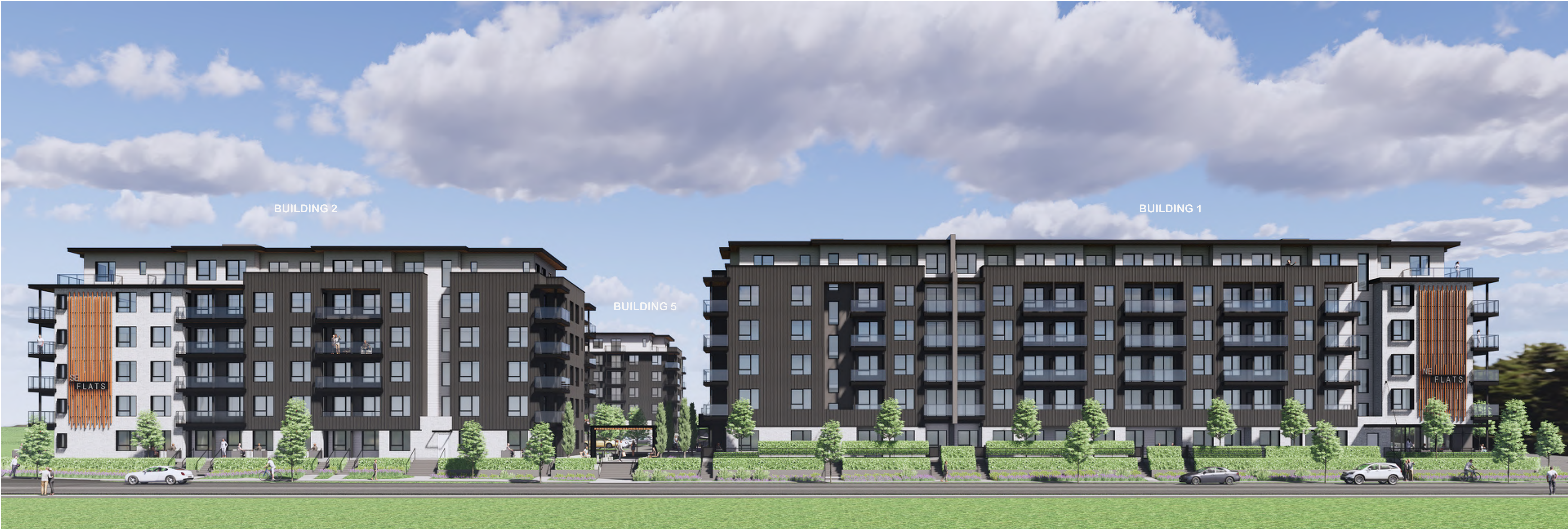
EAST STREETSCAPE VIEW - ALONG 204TH ST.
