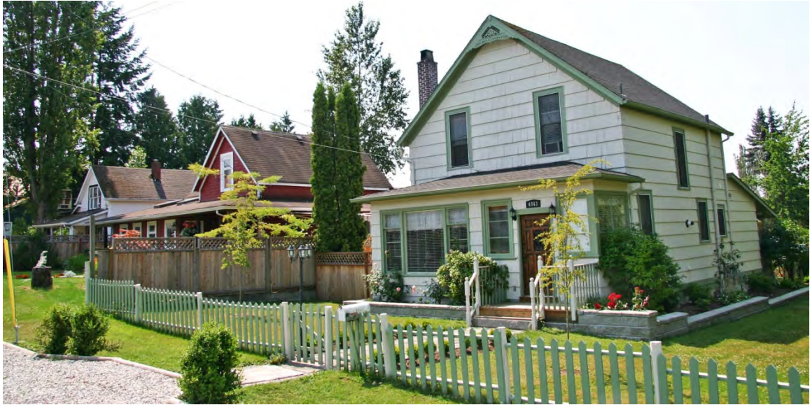
Existing Heritage Streetscape on 216A Street
