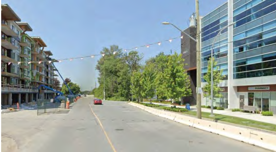
5. Looking to the eastern corner of the site at 86 Avenue
