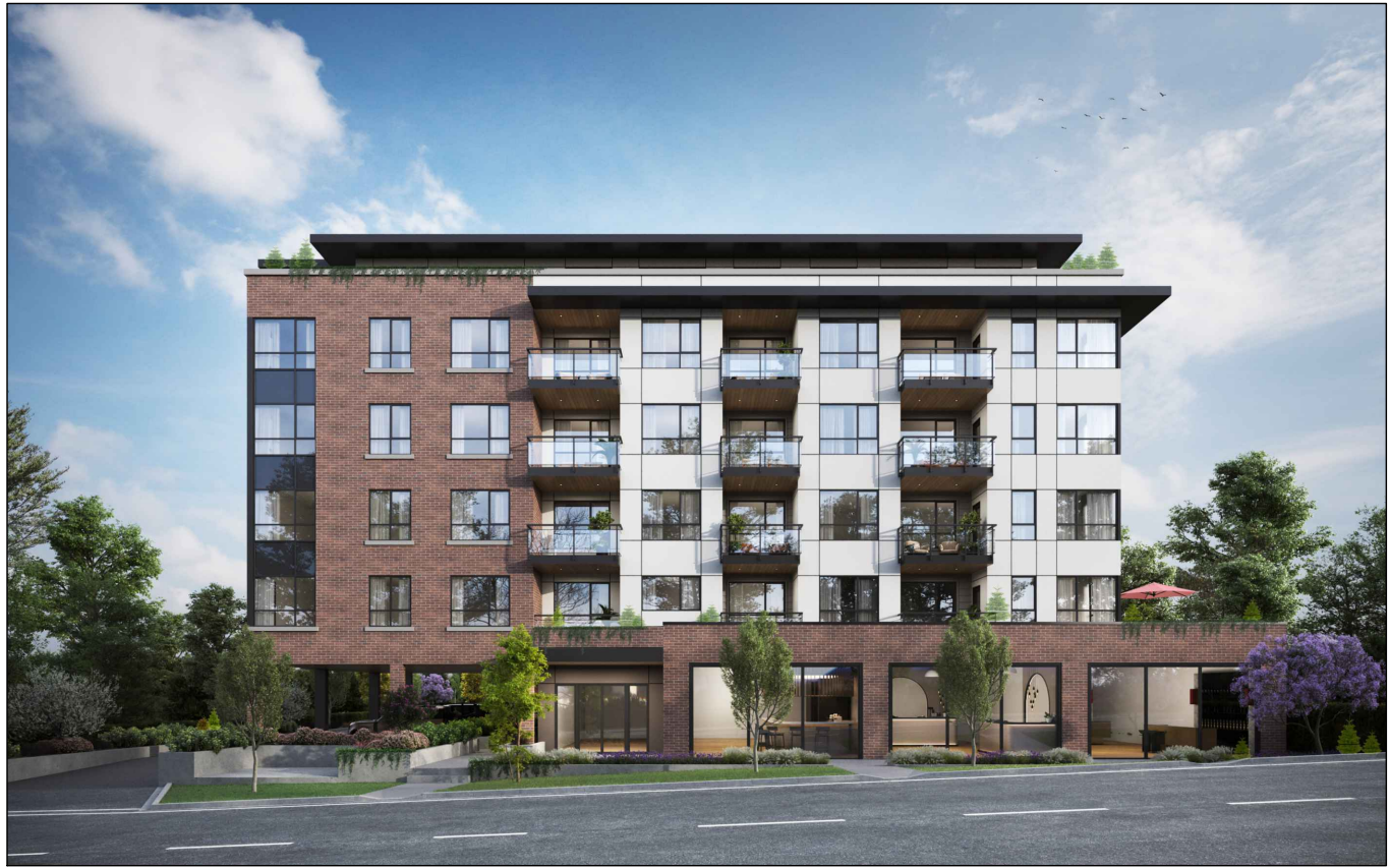
VIEW FROM 82 AVE.
