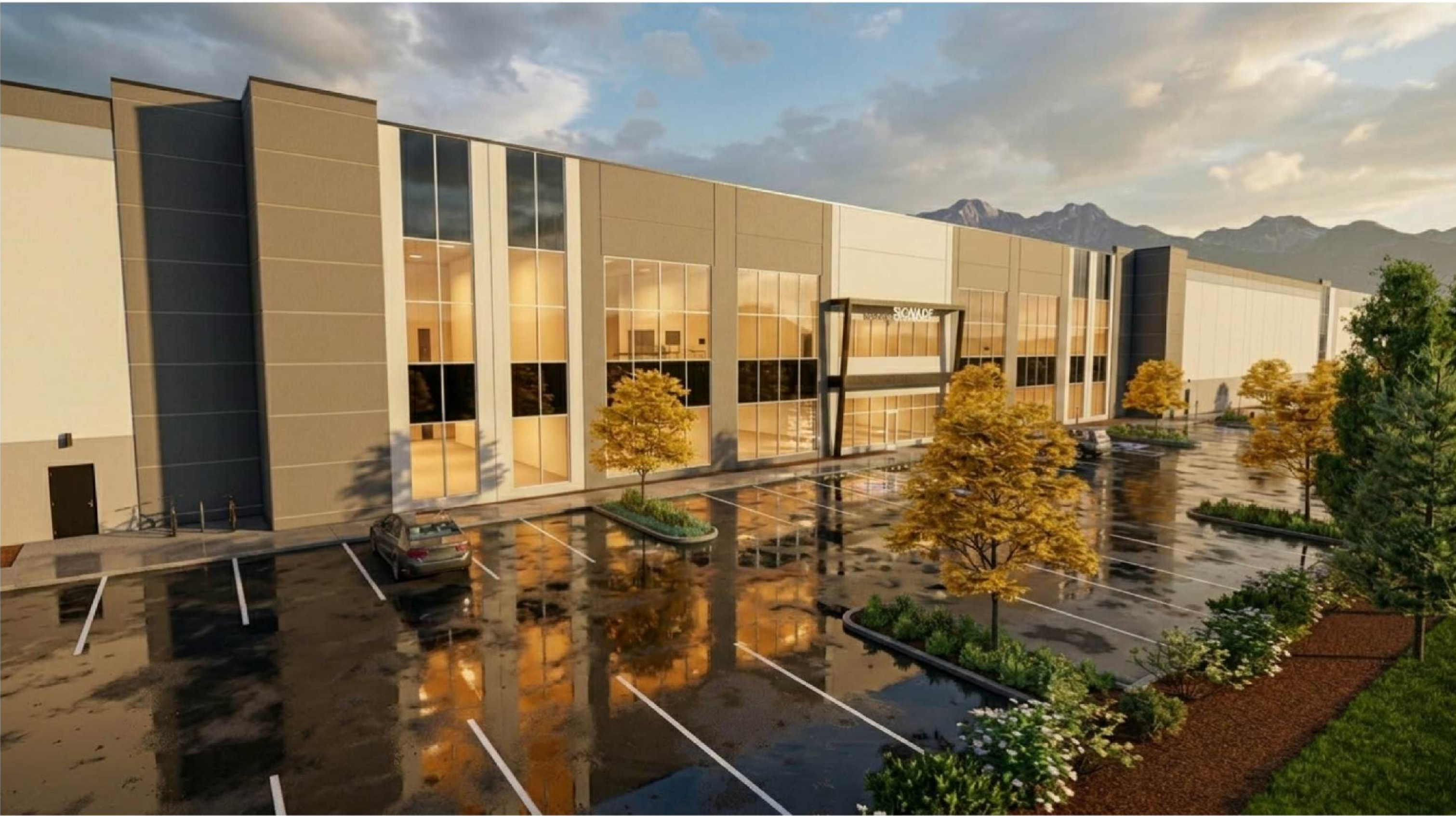
A - Building 1 - Office View
