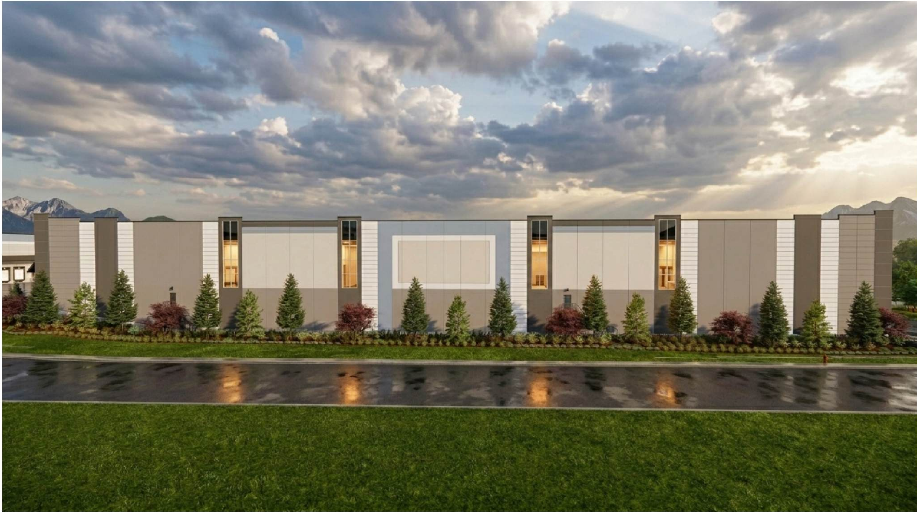
C - Building 2 - South Elevation
