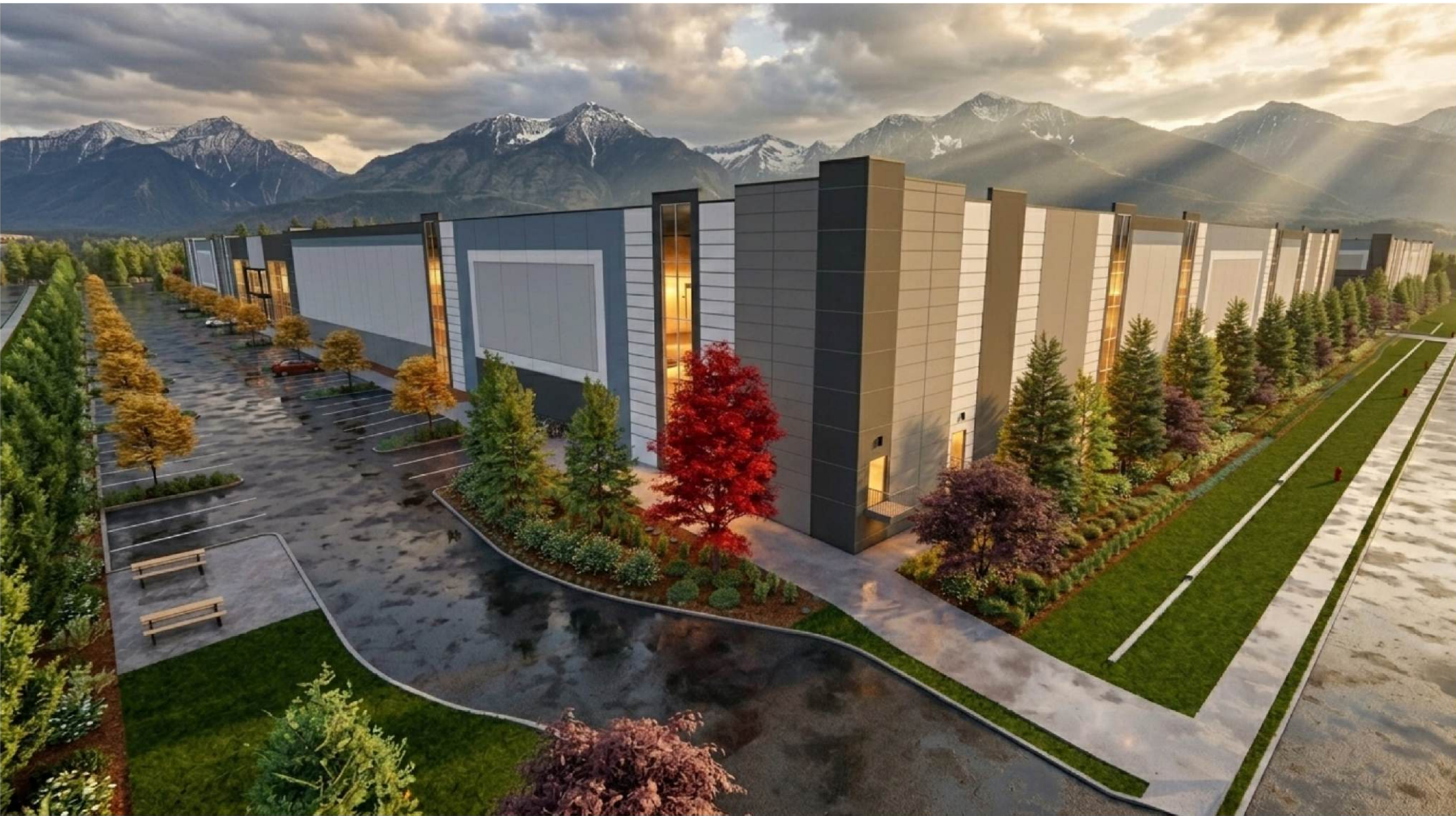
C - Building 1 - South-West View
