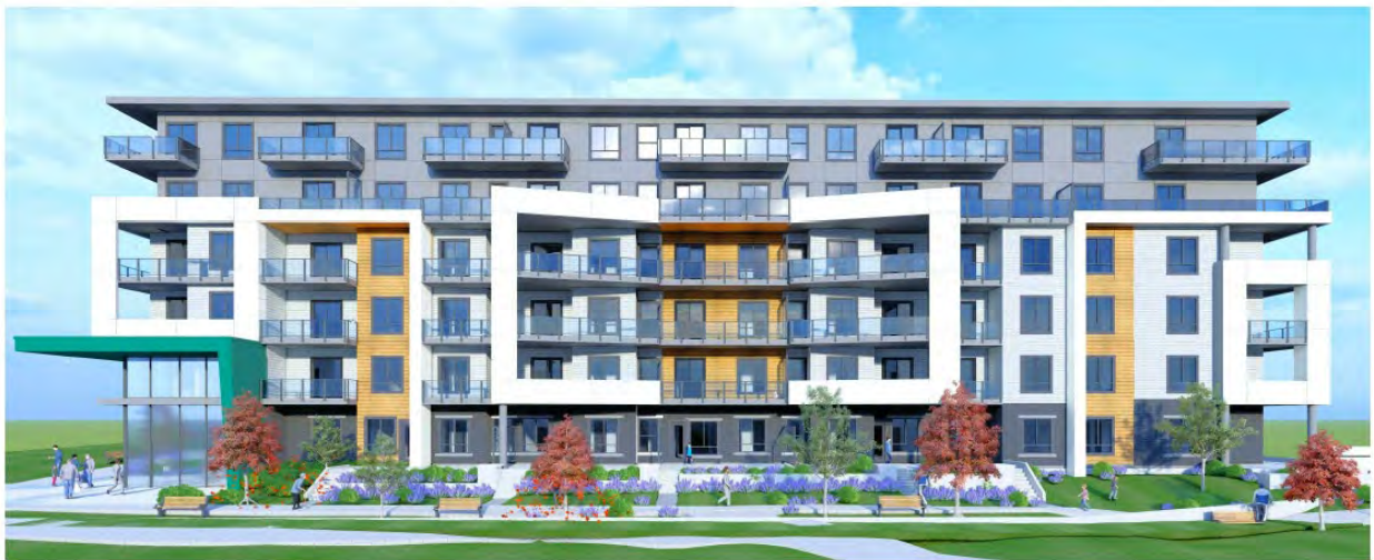
BLDG 2 - WEST VIEW (ENTRANCE SIDE)
