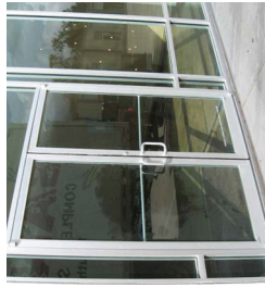
14 STOREFRONT ALUMINUM FRAMED WINDOWS & DOORS CLEAR ANODIZED ALUMINUM & FROSTED TEMPERED GLAZING AT MAIN ENTRANCE LOBBY'S
