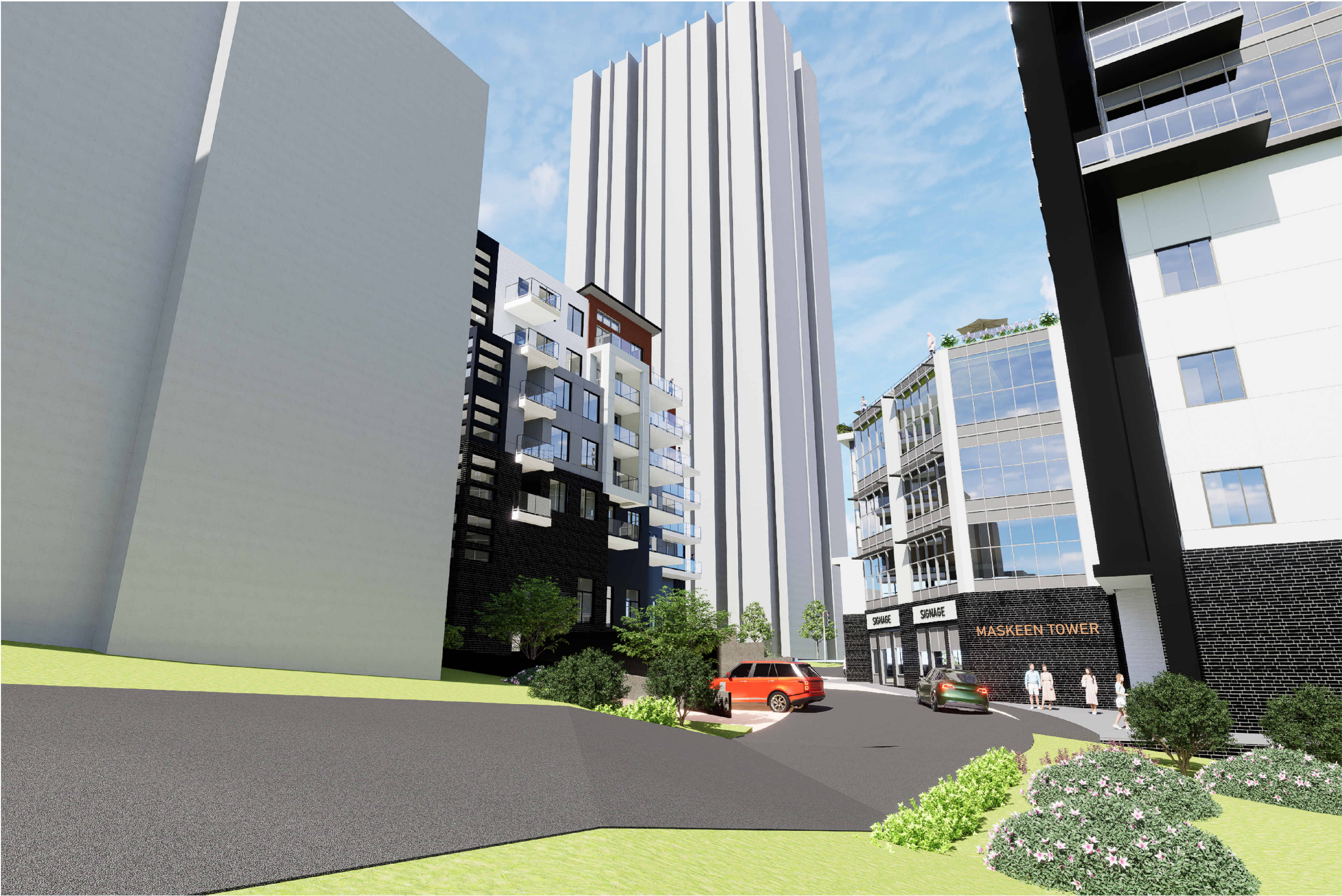
VIEW FROM THE INTERNAL ROAD
