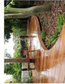
Decking around existing tree
