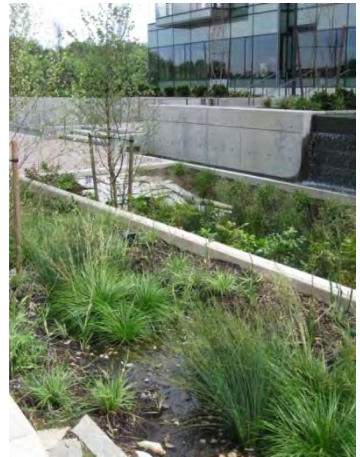
Figure 38. Weirs and check-dams help to slow the flow of water and facilitate infiltration.
