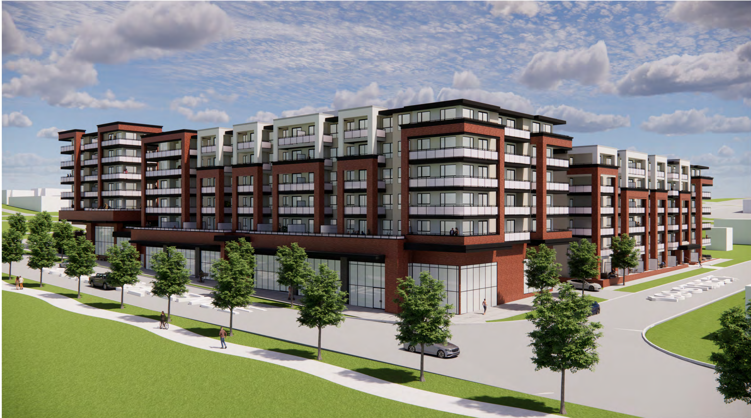
View along 83rd Avenue & 199th Street
