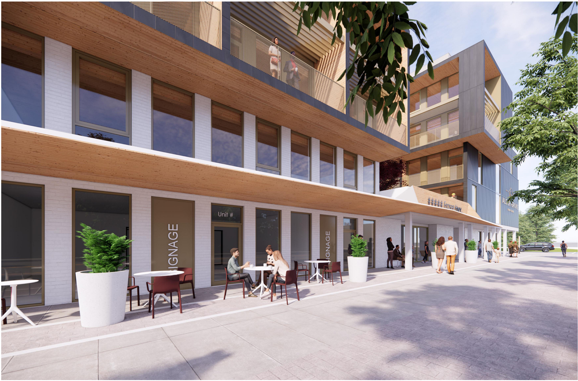
Ground Floor Units along Fraser Highway
