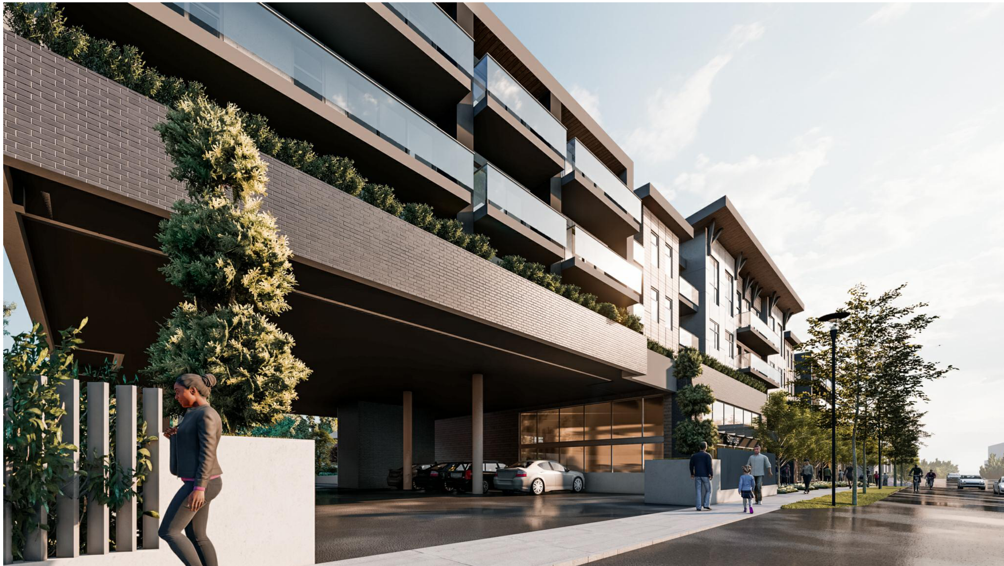
NORTH ELEVATION VIEW OF GROUND FLOOR PARKING AREA
